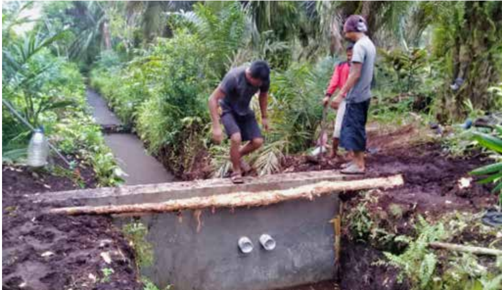
Figure 4.17. Permanent single layer partition wall canal block design agreed with community members
